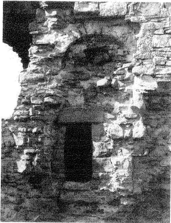
Fig. 3 Tortorwald Castle. Detail of window inserted in original entrance doorway of first floor.
