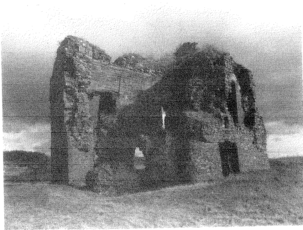
Fig. 4 Torthorwald Castle from N.W., prior to collapse of N.E. corner in 1993.
